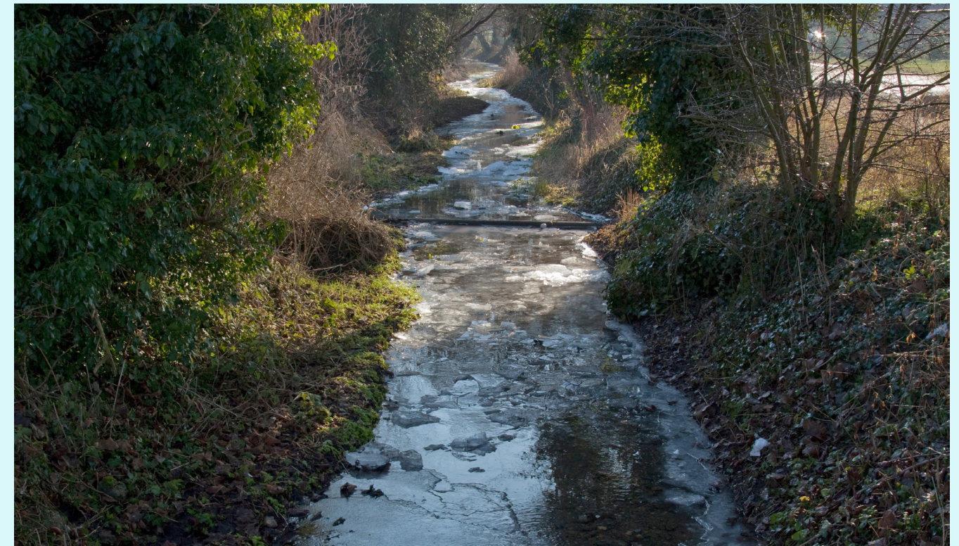
Straightened, over deep channel with steep banks. The channel is disconnected from the floodplain.
