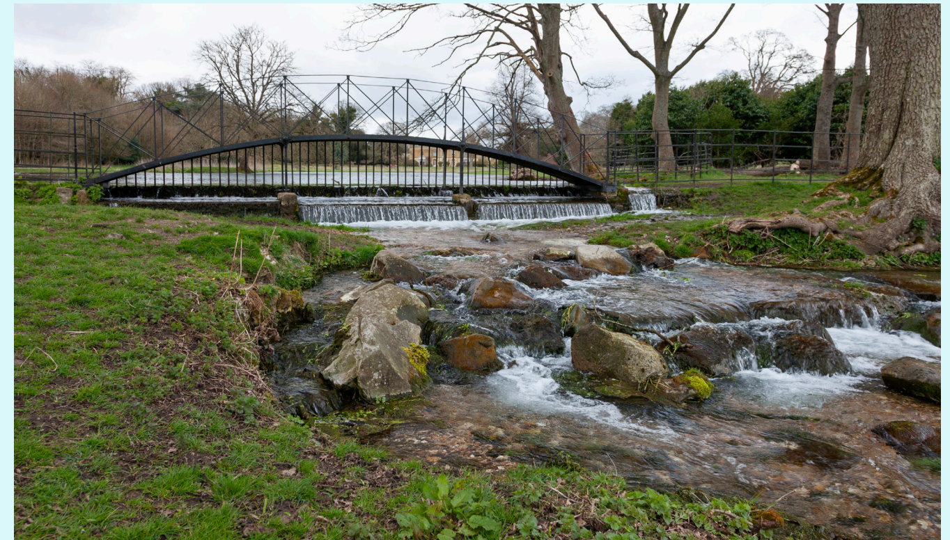
Online pond caused by the weir in the foreground.
